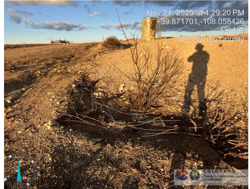
Photo # 4561 Loose barbed wire fencing on location/wildlife hazard
