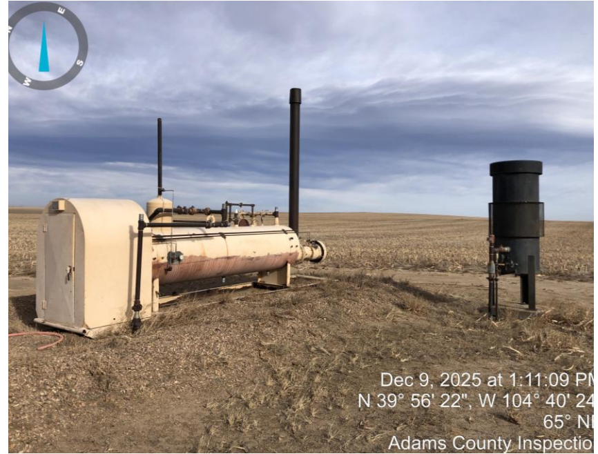
Photo #2 Separator & ECD.
