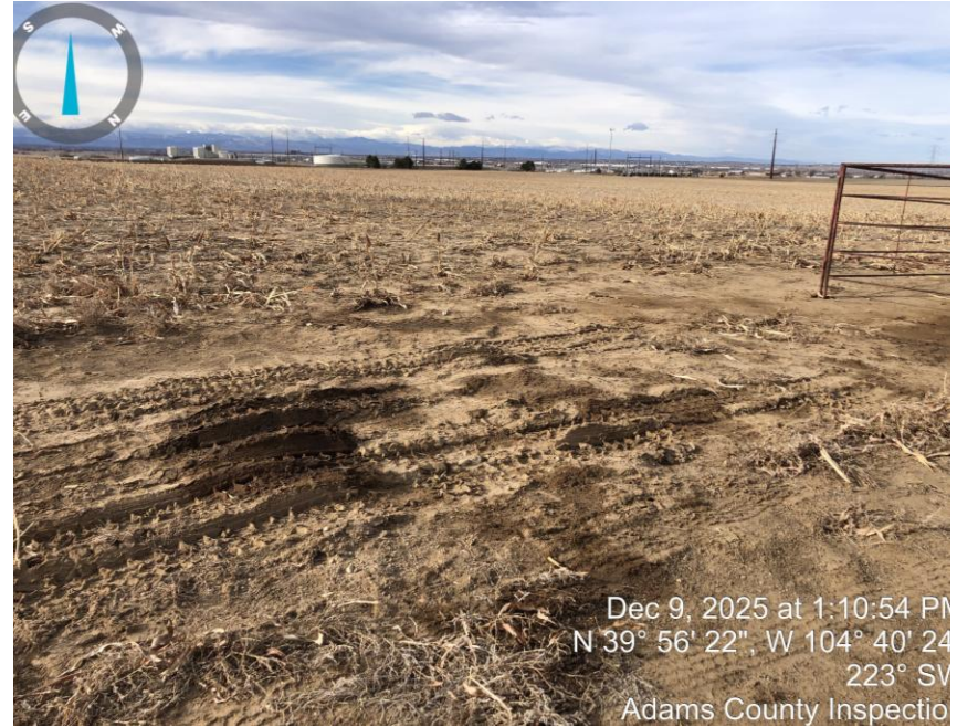
Photo #4 stained soil around the well head.
