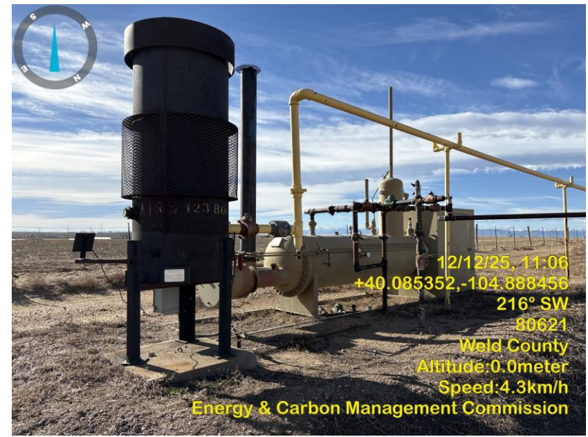
Photo 2 ECD, Horizontal Heated Separator.
