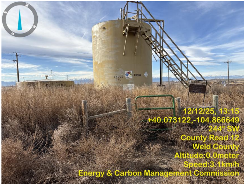
Photo 3 Tank battery overrun with dead vegetation.
