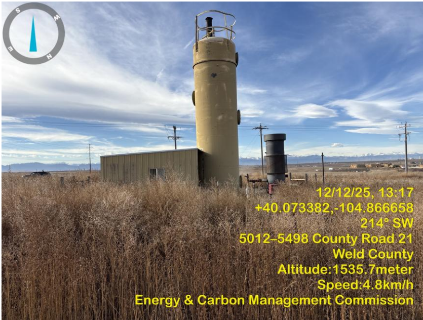
Photo 5 Vertical separator & ECD are overrun with dead vegetation.
