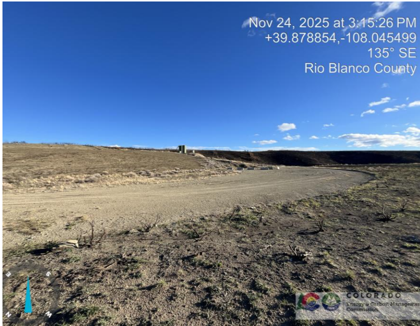
Photo # 4495 NW corner of location
