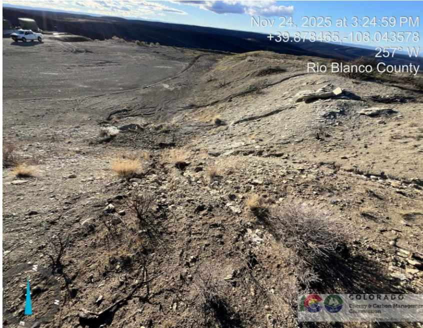
Photo # 4506 Rill erosion & transport of sediment on cut slope/sediment migrating onto location/insufficient BMP's
