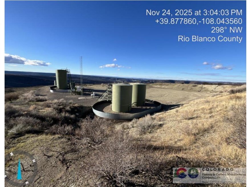
Photo # 4491 SE corner of location
