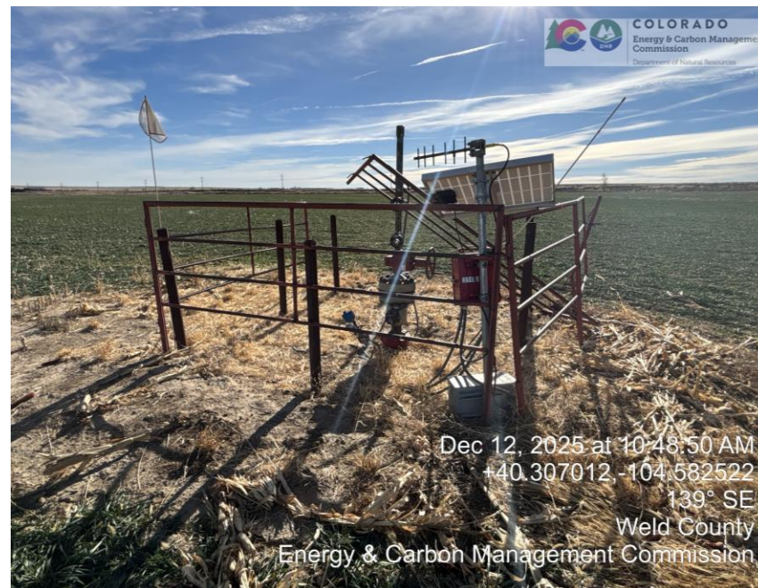
Photo 2 well head and equipment
