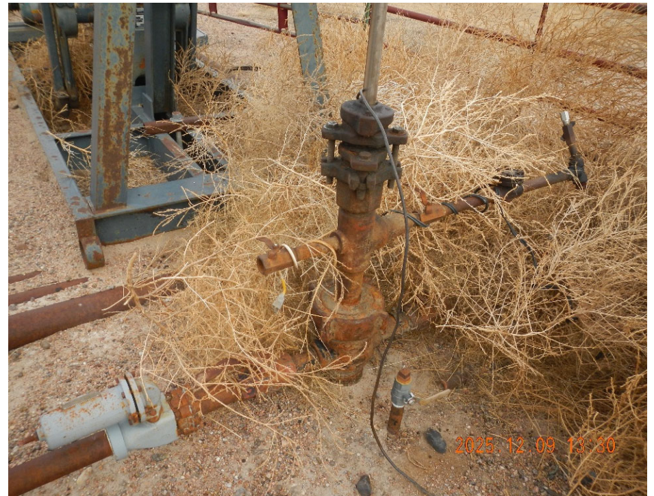
2. View of wellhead.
