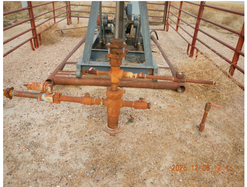
2. View of wellhead.
