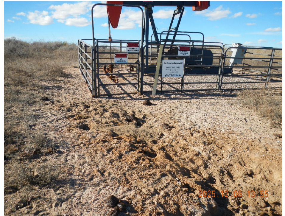
4. View of erosion channel moving down grade looking towards well site.
