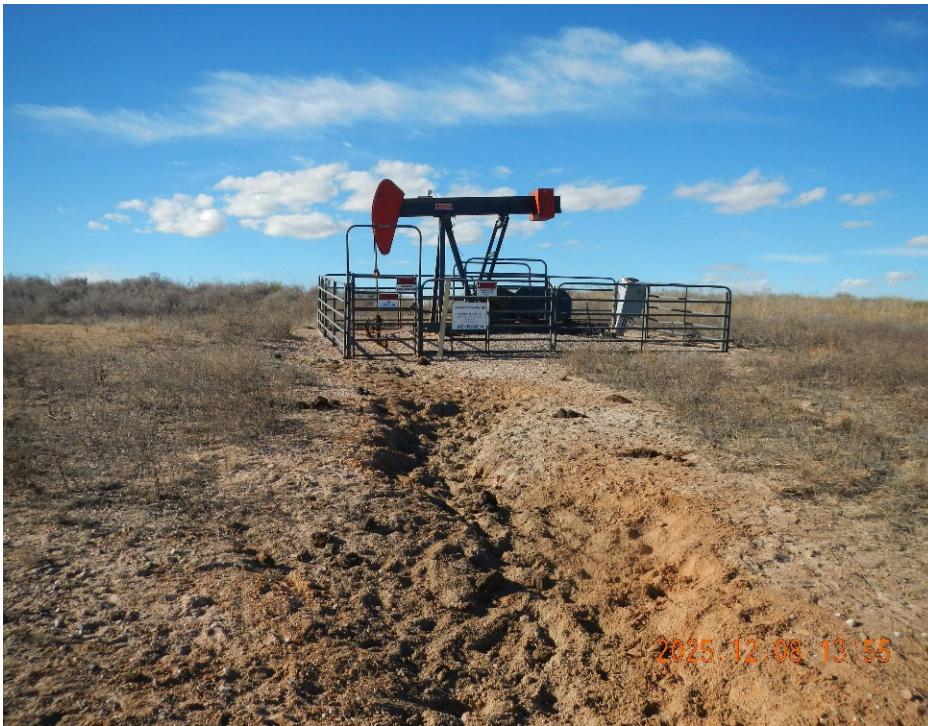
5. View of erosion channel moving down grade looking towards well site.
