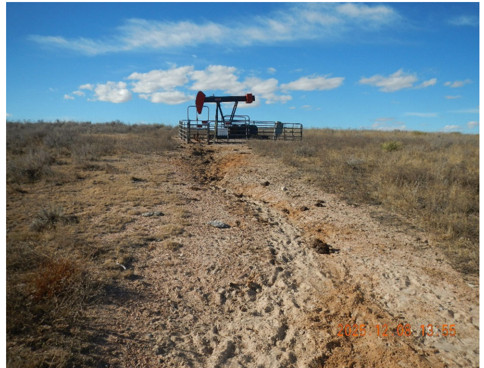
6. View of erosion channel moving down grade looking towards well site.
