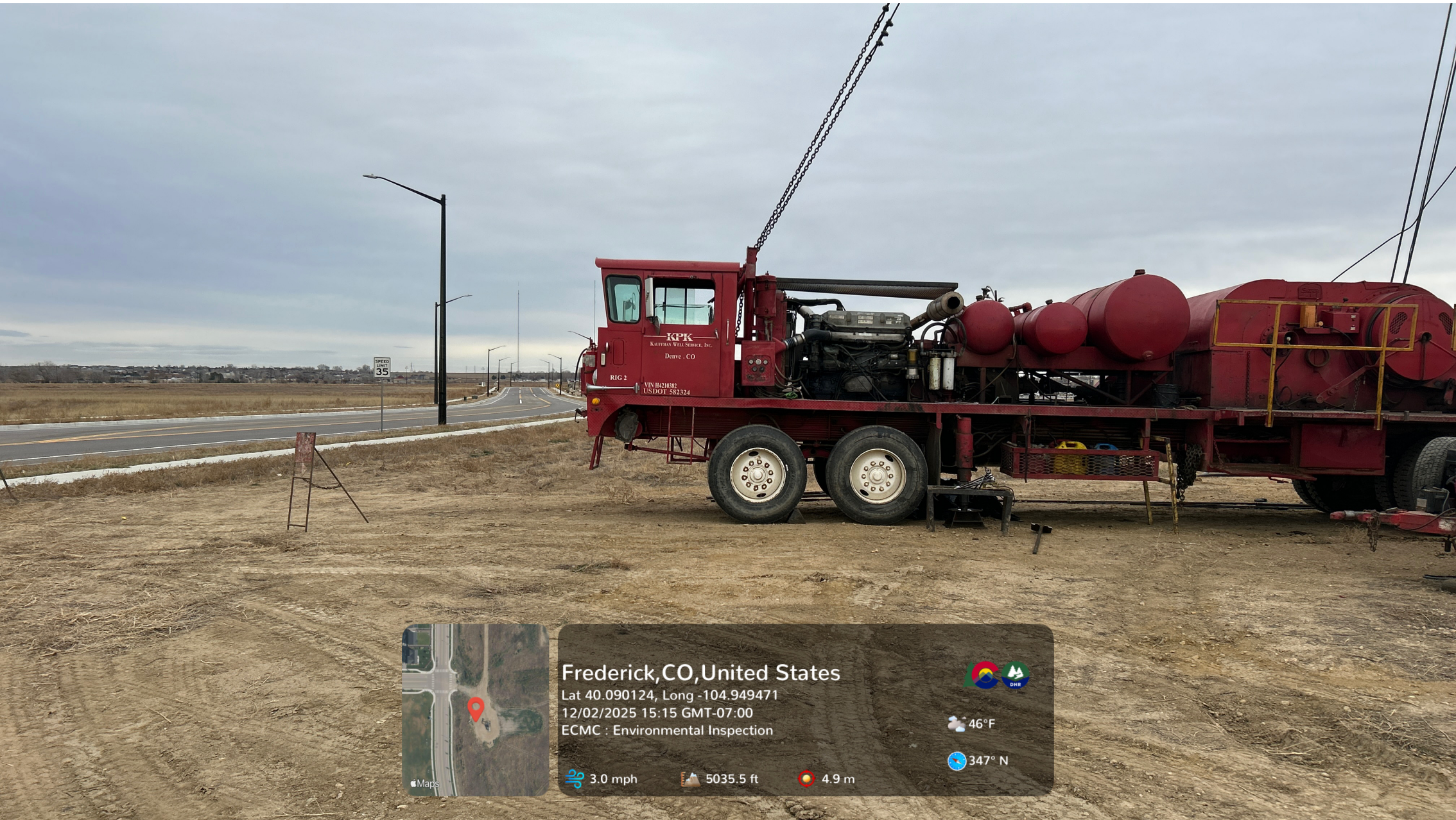
Looking at the workover rig.
