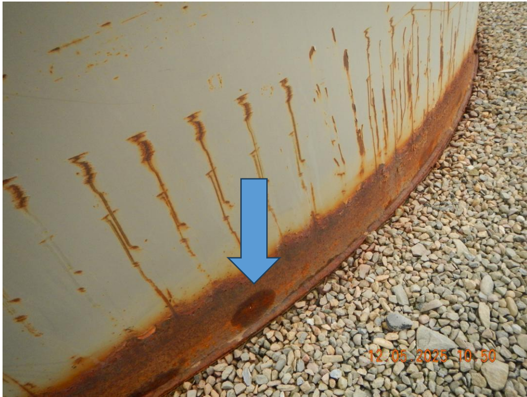
Possible seep starting on tank seam.
