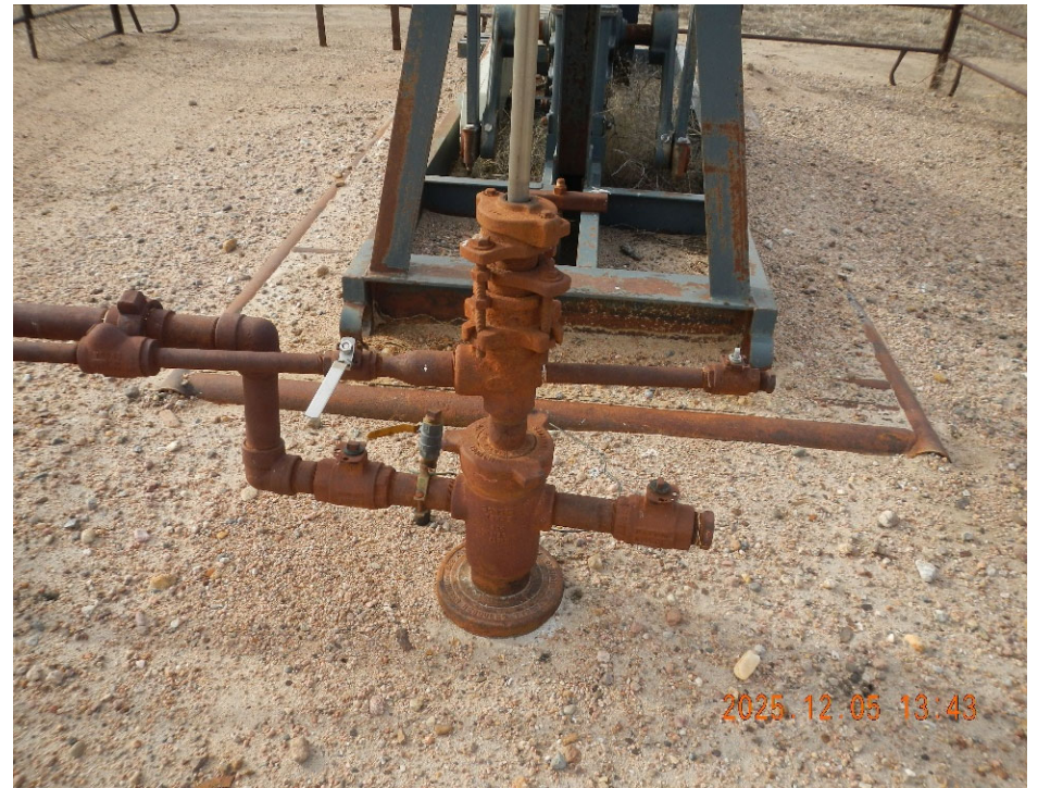
2. View of wellhead.
