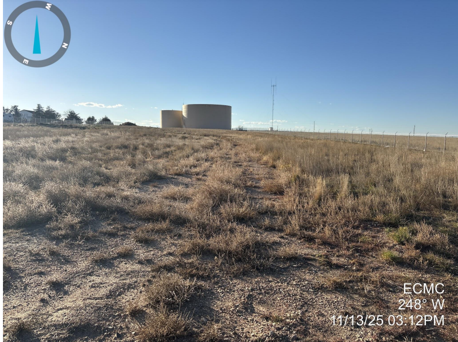
Photo 2. Photo taken of the well location, facing west. See comments under Photo 1.
