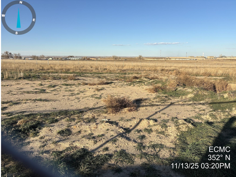
Photo 1. Photo taken of the well location, facing north. Photo illustrates that final reclamation at the location does not meet Rule 1004 standards. The well location is contained within a fenced area.
