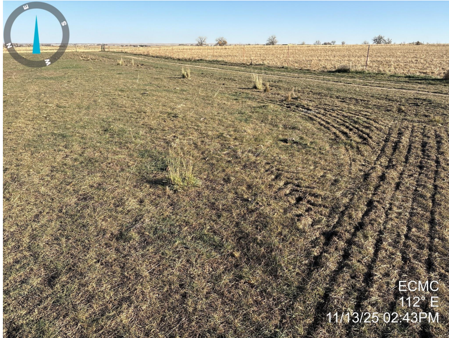
Photo 5. Photo taken of the access road to the well location, facing east. Photo illustrates that vegetation establishment appears to meet Rule 1004 standards.
