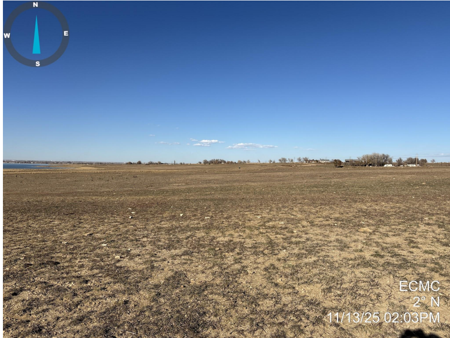
Photo 1. Photo taken of the well location, facing north. Photo illustrates that final reclamation activities have taken place, but vegetation has not established to Rule 1004 standards and gravel was observed across the location.
