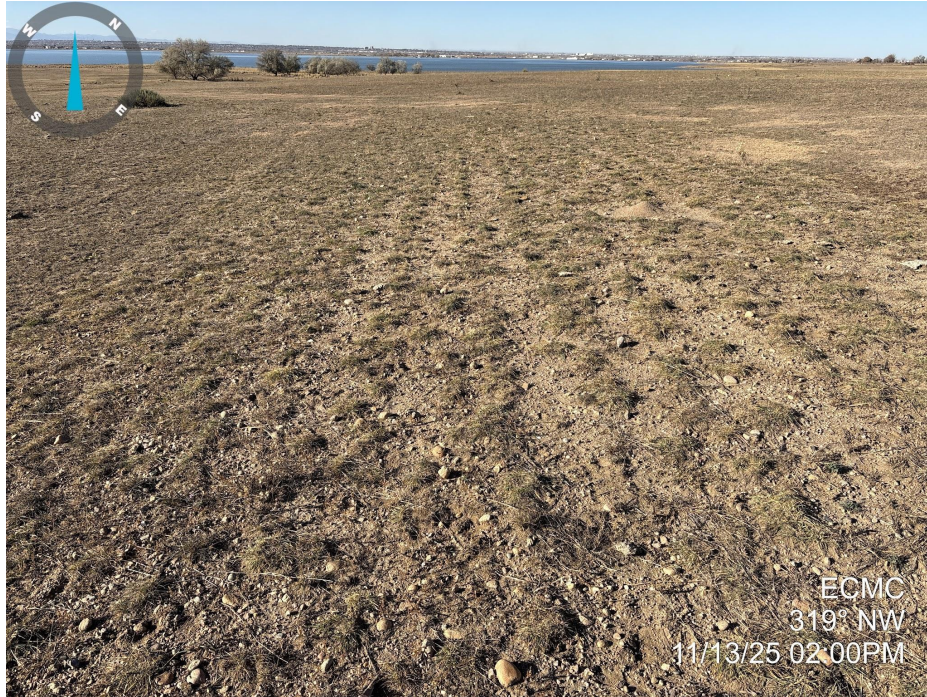
Photo 5. Photo taken of the access road to the location, facing northwest. Photo illustrates that final reclamation activities have taken place, but gravel remains across the access road and vegetation has not established to Rule 1004 standards.
