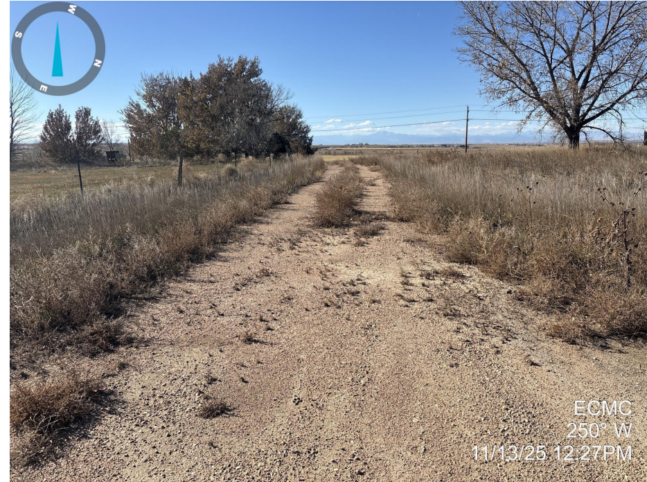
Photo 8. Photo taken of the access road to the location, facing west. Photo illustrates that final reclamation activities have not taken place along the road.
