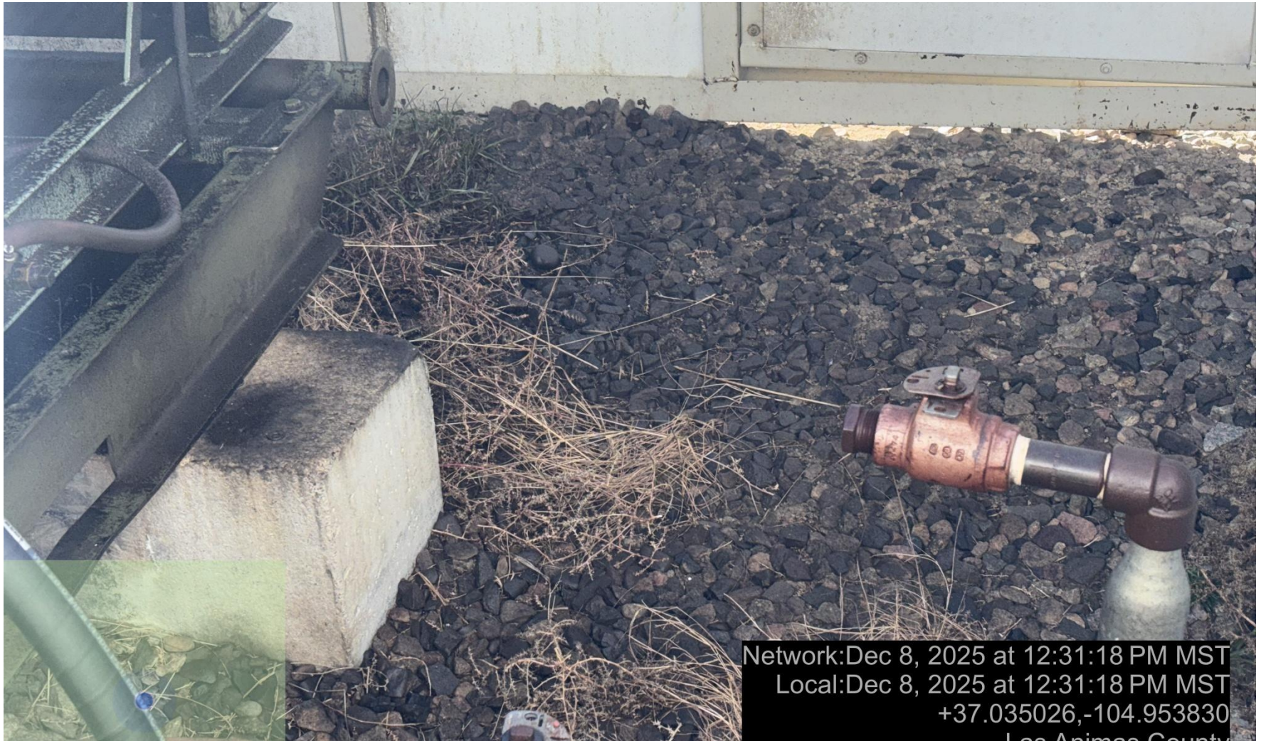
PHOTO 4: IMPACTED OIL NEAR PRIME MOVER SKID. Conduct maintenance on equipment, cleanup stained material and review self inspection processes. COMPLY WITH RULE 1002,(2).D. CA DATE 12-15-2025.
