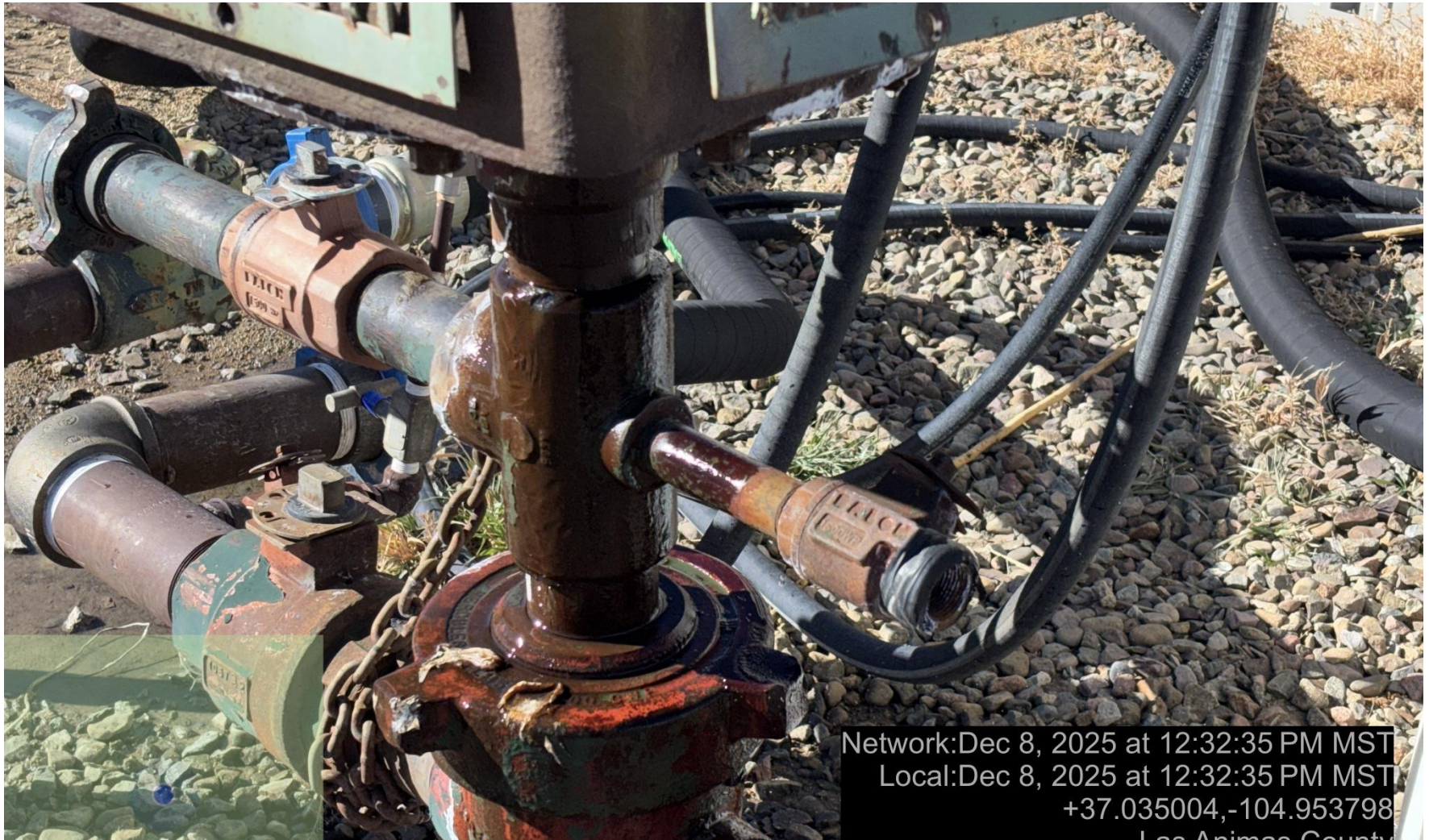
PHOTO 6: PACKING IS LEAKING ON TBG. Securely fasten all valves, pipes, fittings, and Production Facilities to ensure good mechanical condition, inspect at regular intervals and maintain in good mechanical condition. Engineer, operate, and maintain equipment within the manufacturer's recommended specifications per Rule 608.e. CA DATE 12-9-2025.
