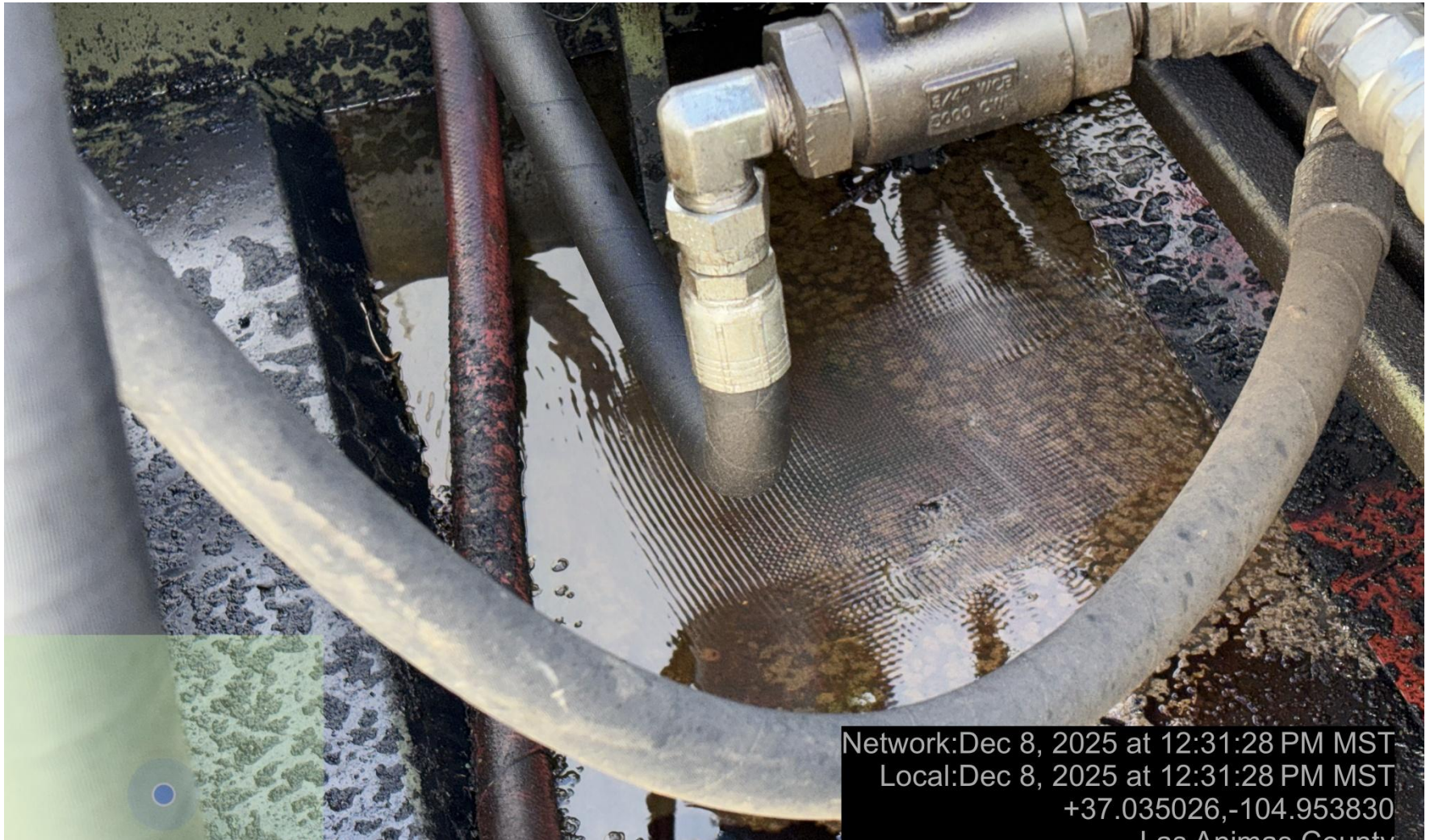
PHOTO 8: OILY WASTE IS PRIME MOVER SKID. DRAIN OILY WASTE REPAIR ALL LEAKS AND REMOVE IMPACTED SOIL PER RULE 1002.(2).D & 1002.f.(2)B, Comply with general provisions of the oil and gas act for wildlife protection AND SB-181. CA DATE 12-9-2025.
