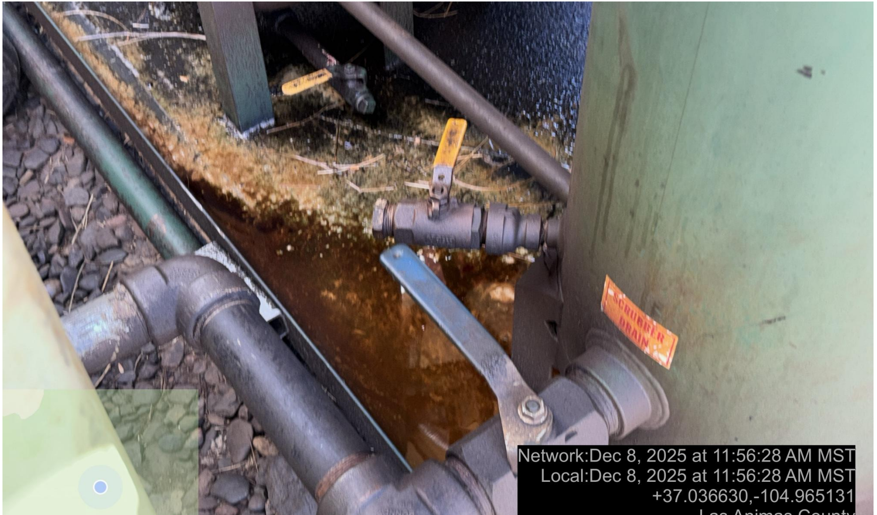
PHOTO 6: OILY WASTE IN COMPRESSOR SKID. DRAIN OILY WASTE REPAIR ALL LEAKS AND REMOVE IMPACTED SOIL PER RULE 1002..(2).D & 1002.f.(2)B, Comply with general provisions of the oil and gas act for wildlife protection AND SB-181. CA DATE 12-9-2025.
