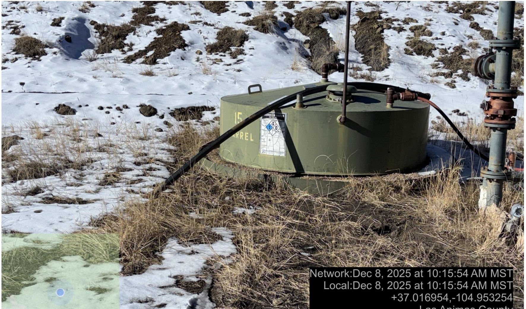
PHOTO 4: UNUSED EQUIPMENT (2" POLY PIPE ON 15 BBL TANK). REMOVE UNUSED EQUIPMENT PER RULE 606. CA DATE 12-15-2025.
