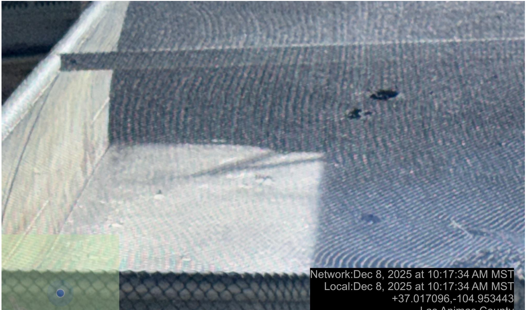
PHOTO 5: Netting on open top tanks inadequate. Install or repair wildlife protection equipment per rule 608.a.(13). CA DATE 12-15-2025.
