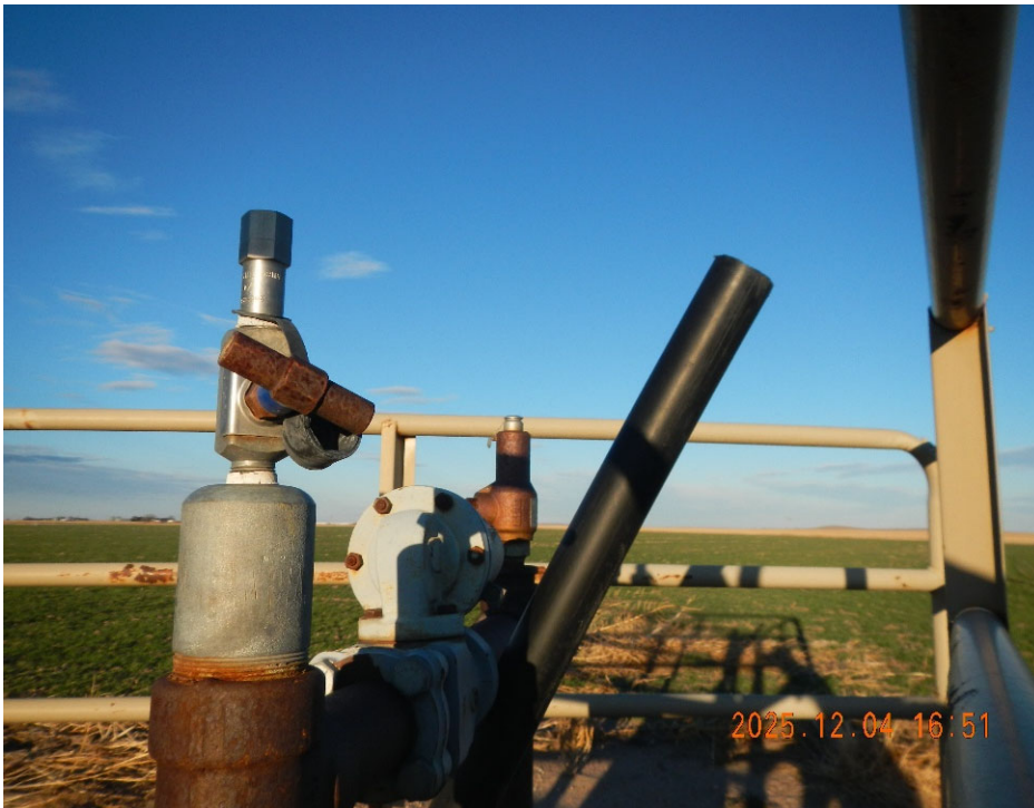
9. View of open ended stubbed up poly pipe at well location.
