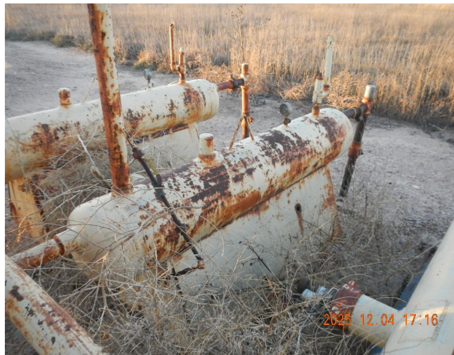
6. Horizontal separator at remote gathering location.
