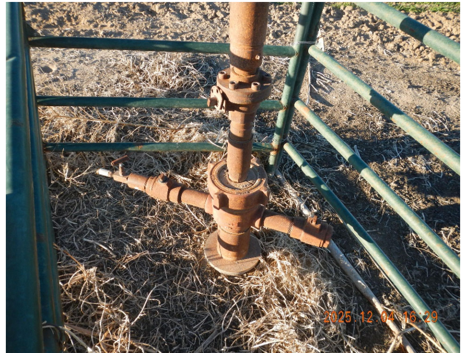
2. View of wellhead. Note Bradenhead not visible at surface.
