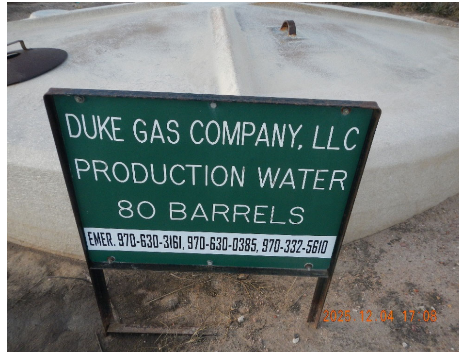
6. View of produced water tank sign at remote gathering location. Note sign missing NFPA label.
