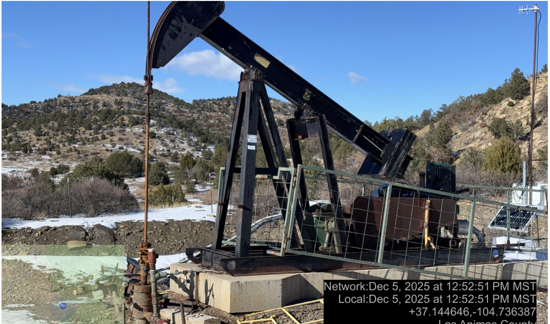
PHOTO 3: WELLHEAD AND EQUIPMENT.
