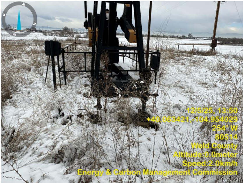
Photo 5 Tall dead vegetation around the wellhead is snow covered.
