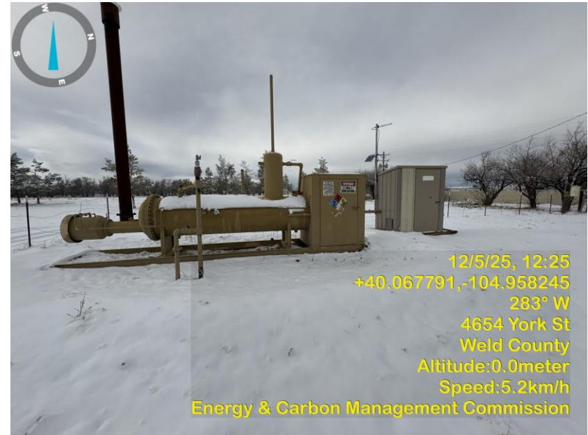
Photo 2 Horizontal Heated Separator, Gas Meter Run.
