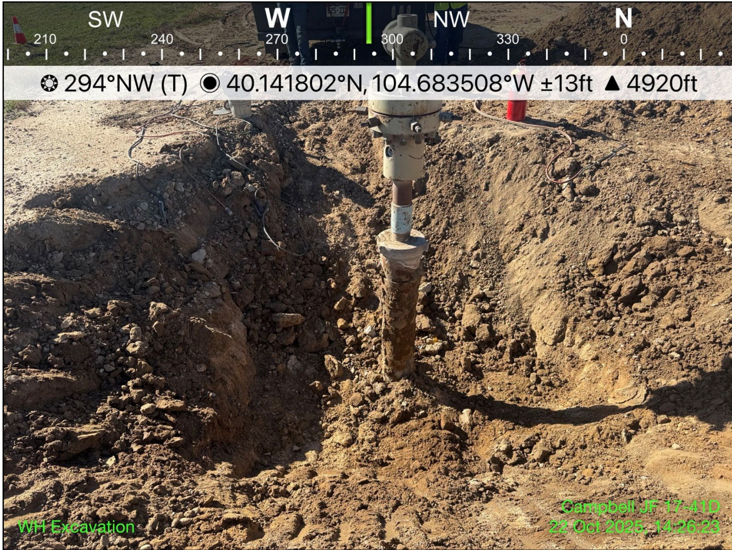
Photo 3: View of wellhead excavation, facing west-northwest
