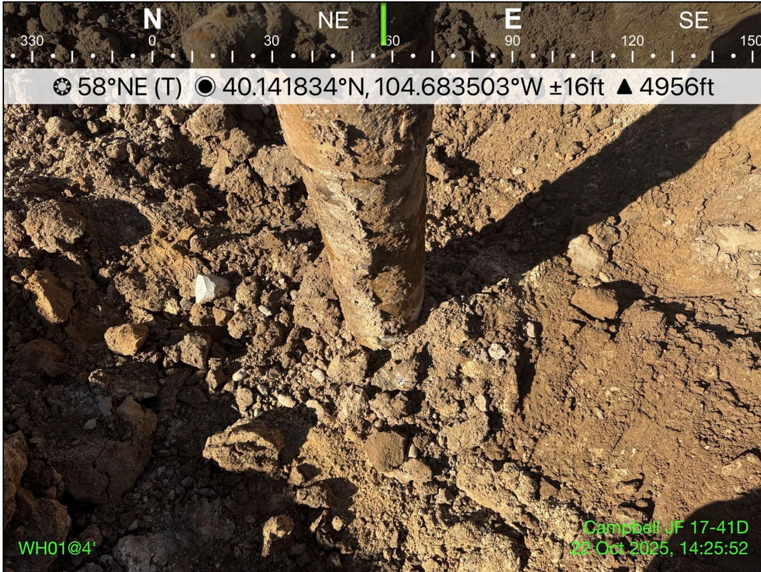
Photo 1: View of wellhead excavation, facing northeast
