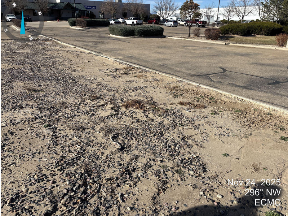
Photo 3. Looking west down the north side of the location. Sediment appears to be moving to this area of the location through stormwater erosion.
