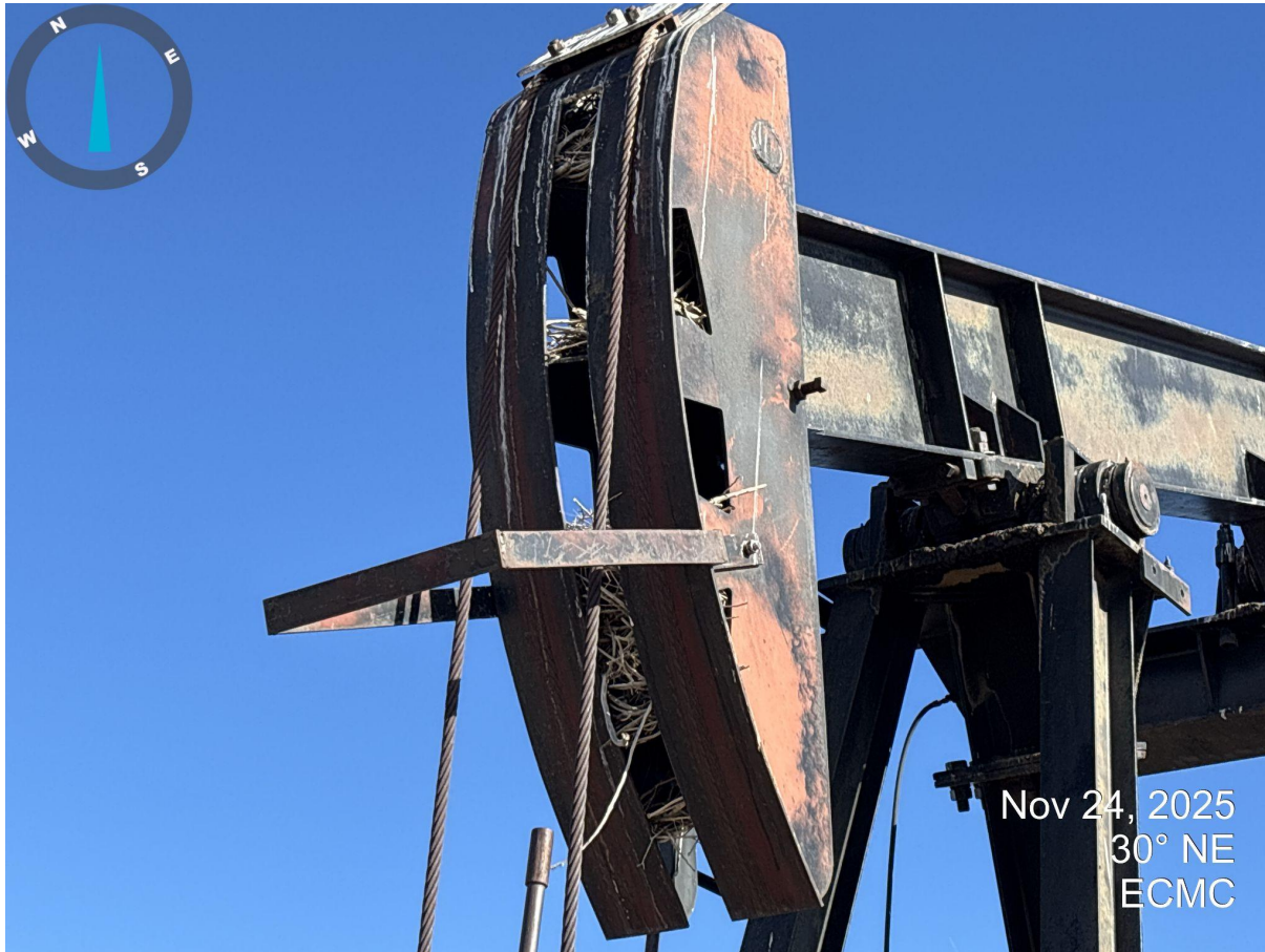
Photo 5. Bird nesting material/ debris is present in the pumpjack head.
