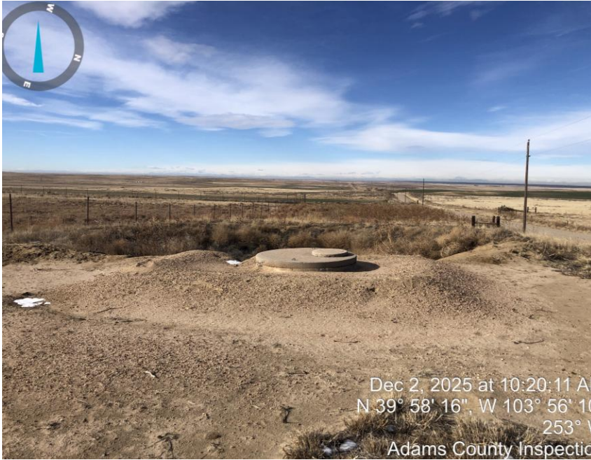
Photo #3 Vault & pit.
