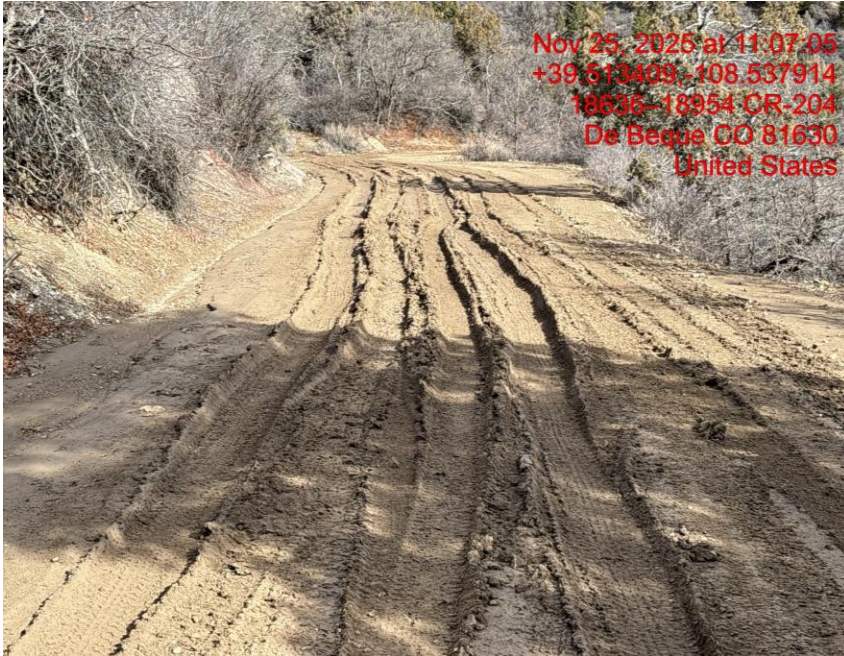
Lack of Stabilization/Insufficient Erosion Controls on Lease Road – Photo #01775
