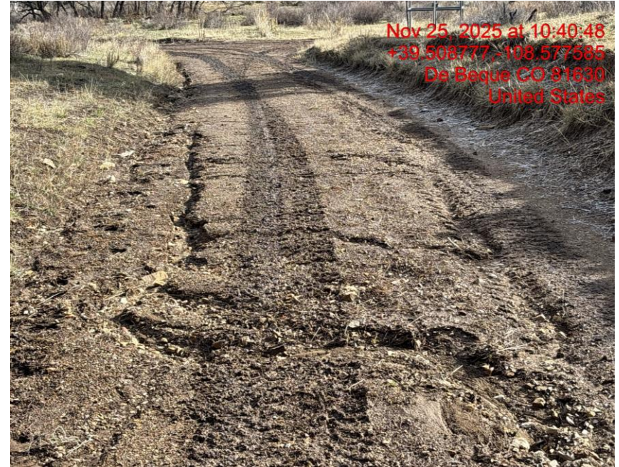
Insufficient Erosion Controls on Lease Road – Photo #01745
