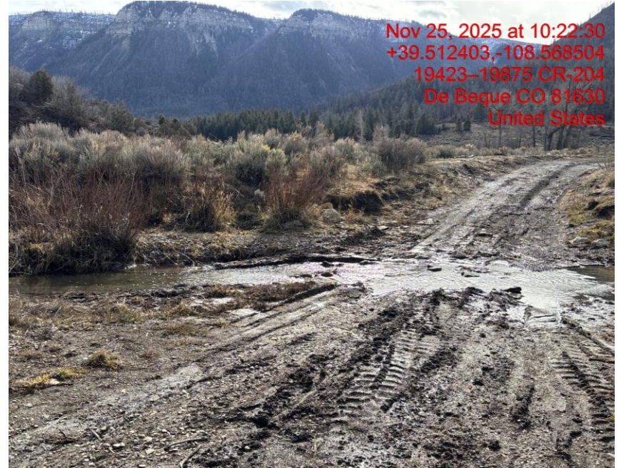
No BMPs or Erosion Controls at Stream Crossing – Photo #01732
