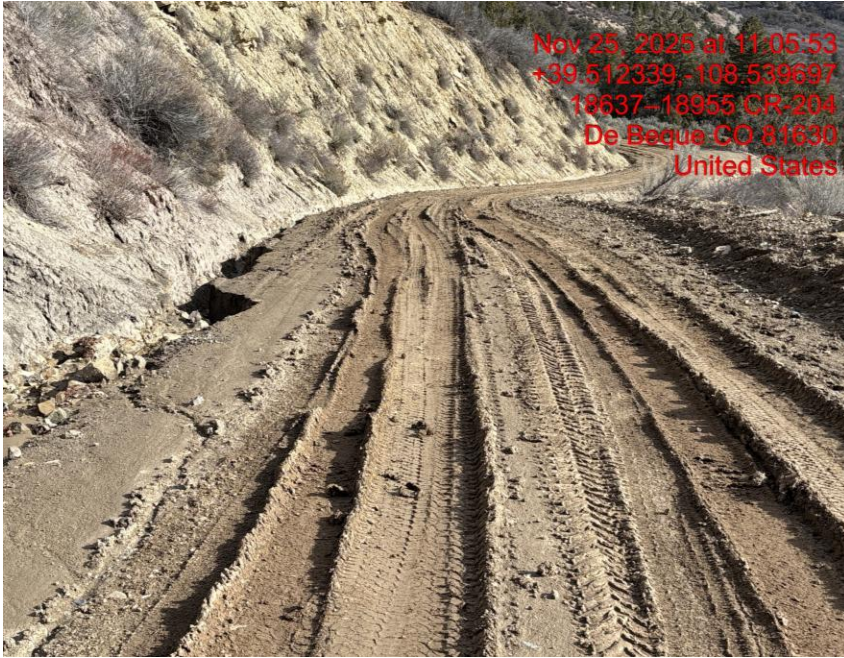
Lack of Stabilization on Lease Road – Photo #01774
