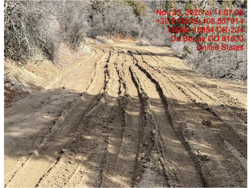
Lack of Stabilization on Lease Road – Photo #01775
