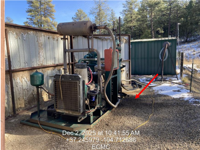
Photo 5 – Stained soils at base of engine skid
