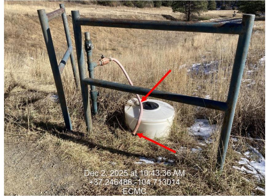
Photo 6 – Red hose not properly secured in tank
