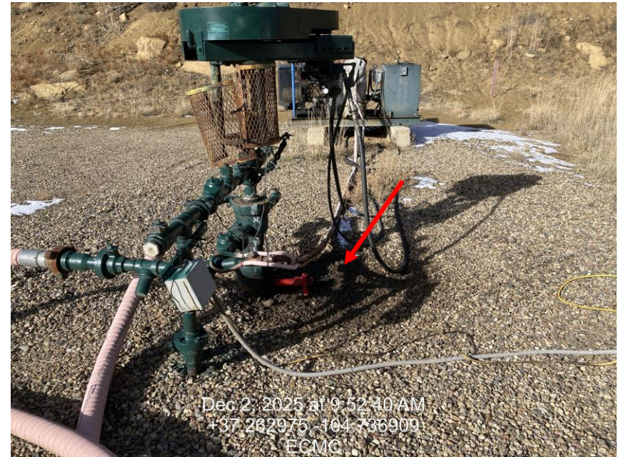
Photo 4 – Stained soils at base of wellhead
