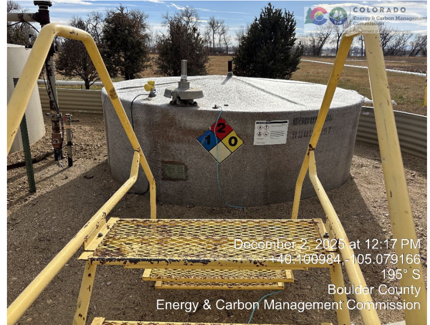
Produced water tank placards
