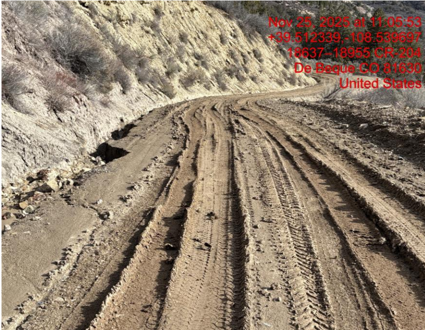
Lack of Stabilization on Lease Road – Photo #01774
