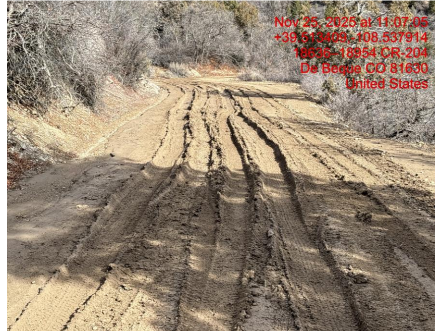
Lack of Stabilization on Lease Road – Photo #01775
