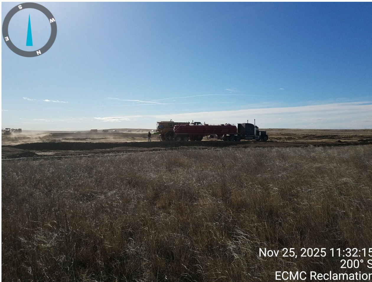
Photo 3. Photo taken of the northwestern location, facing South. Photo illustrates a water supply truck filling up the watering truck used for dust mitigation.
