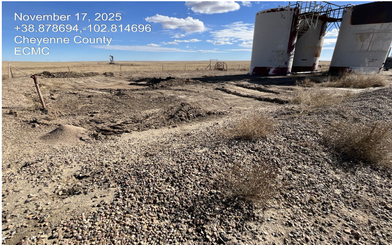
Photo 1. Facing southeast toward the tank battery. The E&P waste stored at this area was removed however there is still a pile of loose material that could be remnants leftover.
