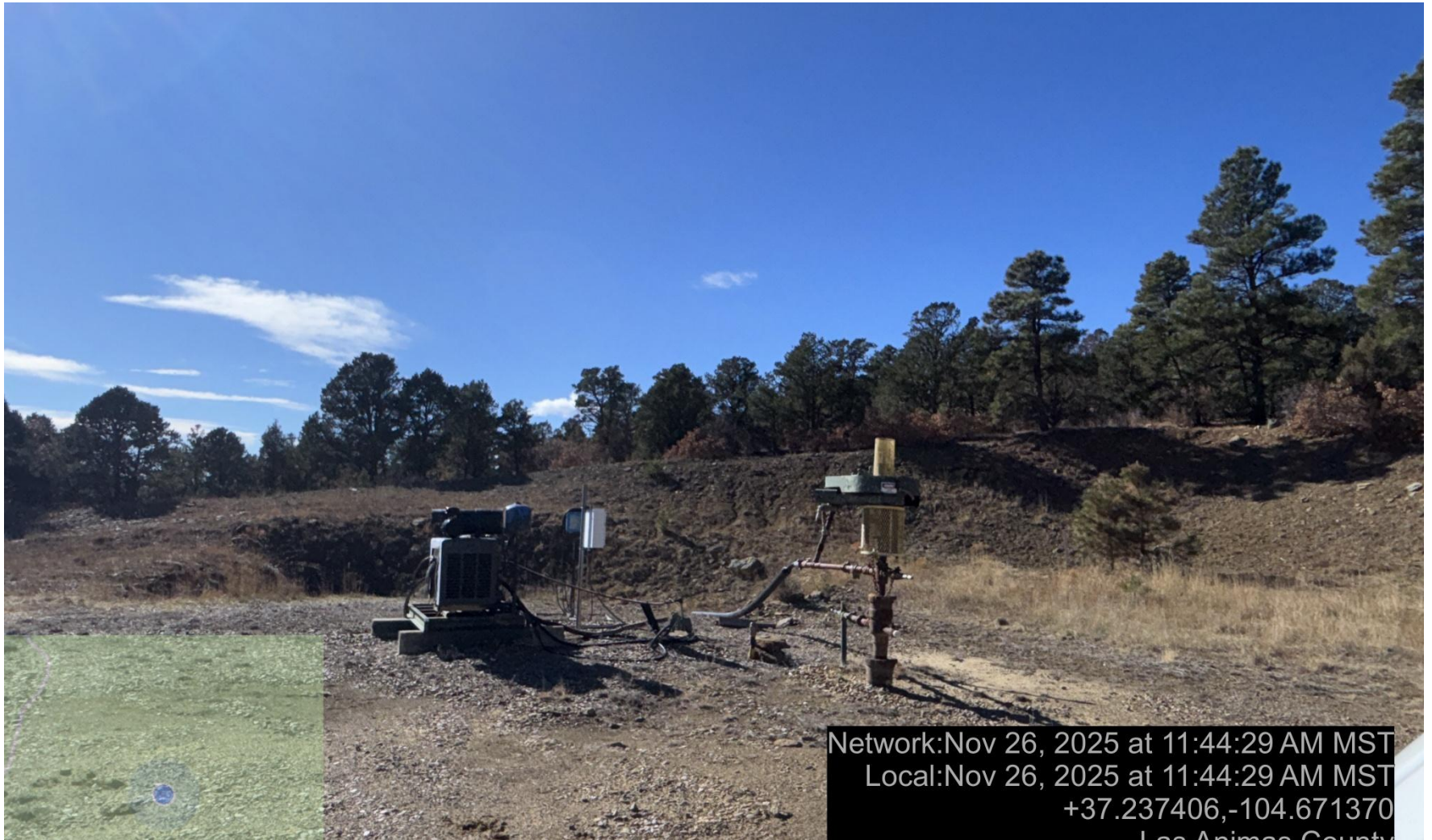
PHOTO 3: WELLHEAD AND EQUIPMENT.
