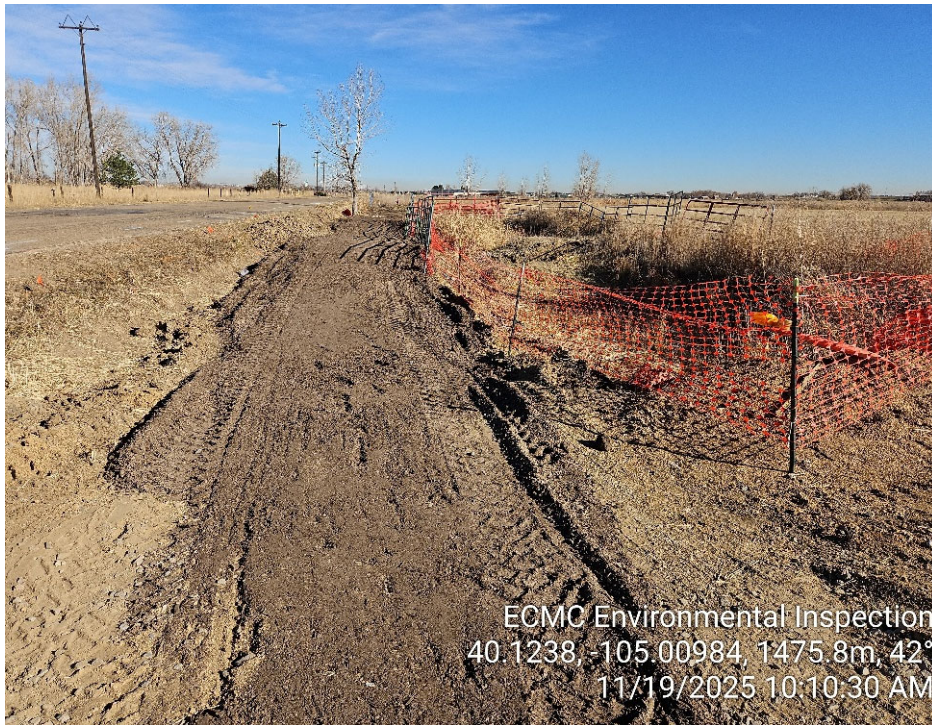
Photo 9 – Backfilled area west of excavation
