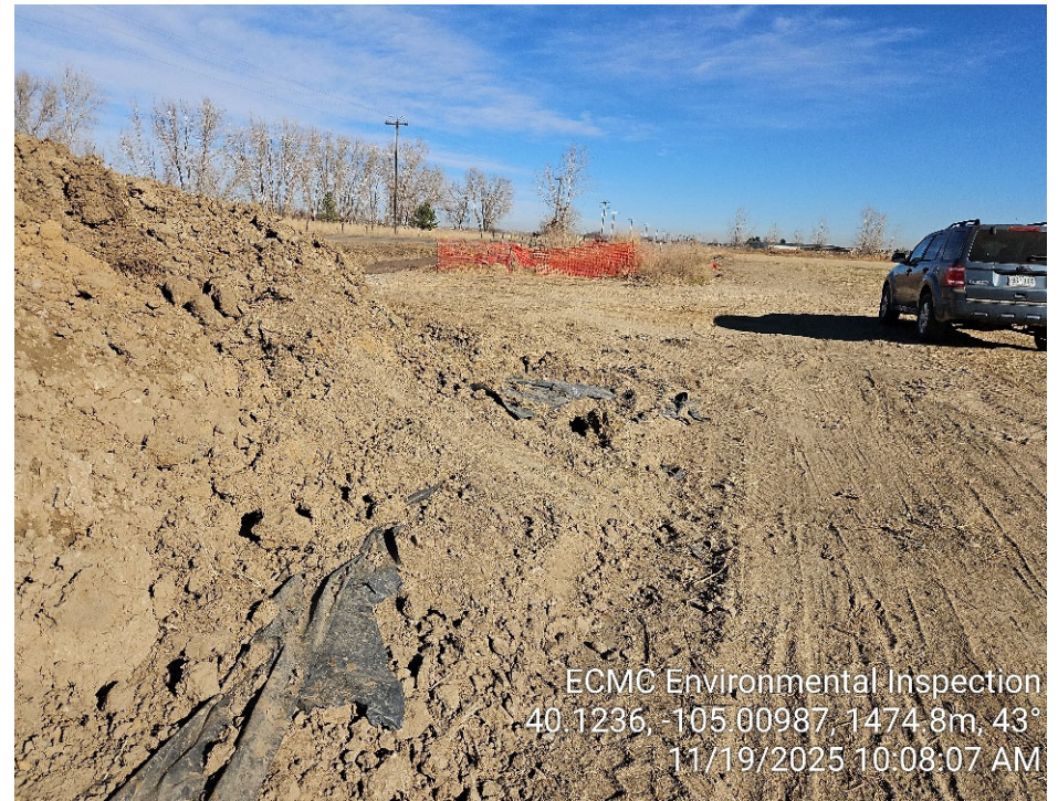
Photo 14 - Soil stockpile. Liner is torn. Stormwater BMPs missing/inadequate.
