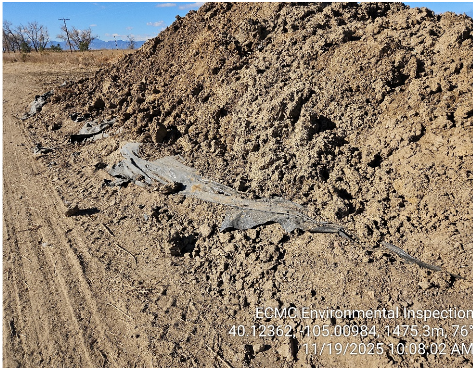
Photo 13 – Soil stockpile. Liner is torn. Stormwater BMPs missing/inadequate.
