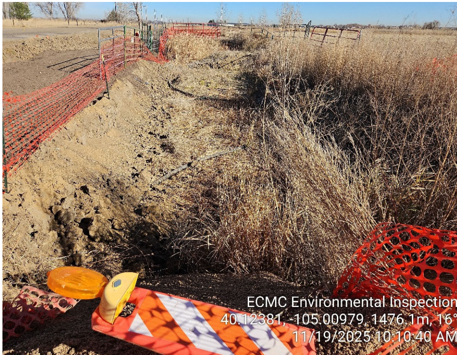
Photo 5 – Open excavation. No groundwater currently present.
