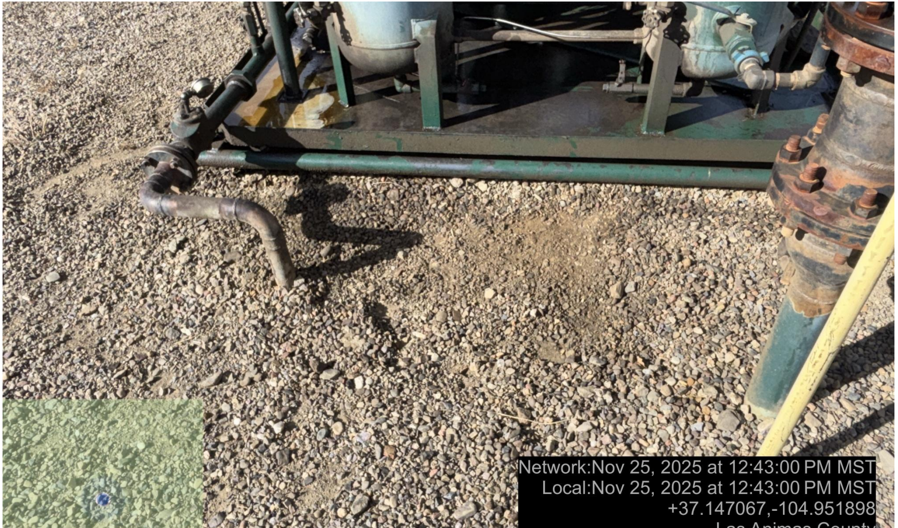
PHOTO 4: Impacted soil identified near compressor skid. Conduct maintenance on equipment, cleanup stained material and review self inspection processes. COMPLY WITH RULE 1002,(2).D. this is the 2 nd notice for this corrective action, immediate action is required.
