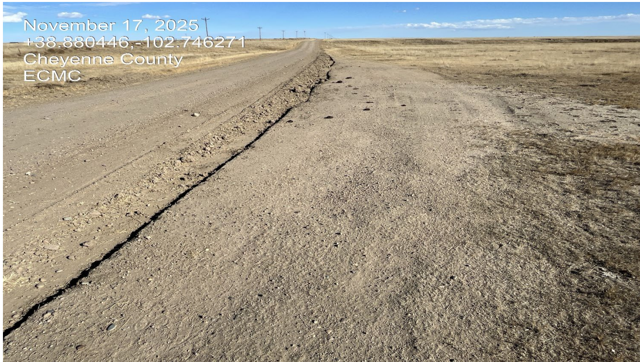
Photo 2. Facing east along the access road. The road has been regraded. This disturbed area where vehicles were driving will need to be decompacted and reclaimed.
