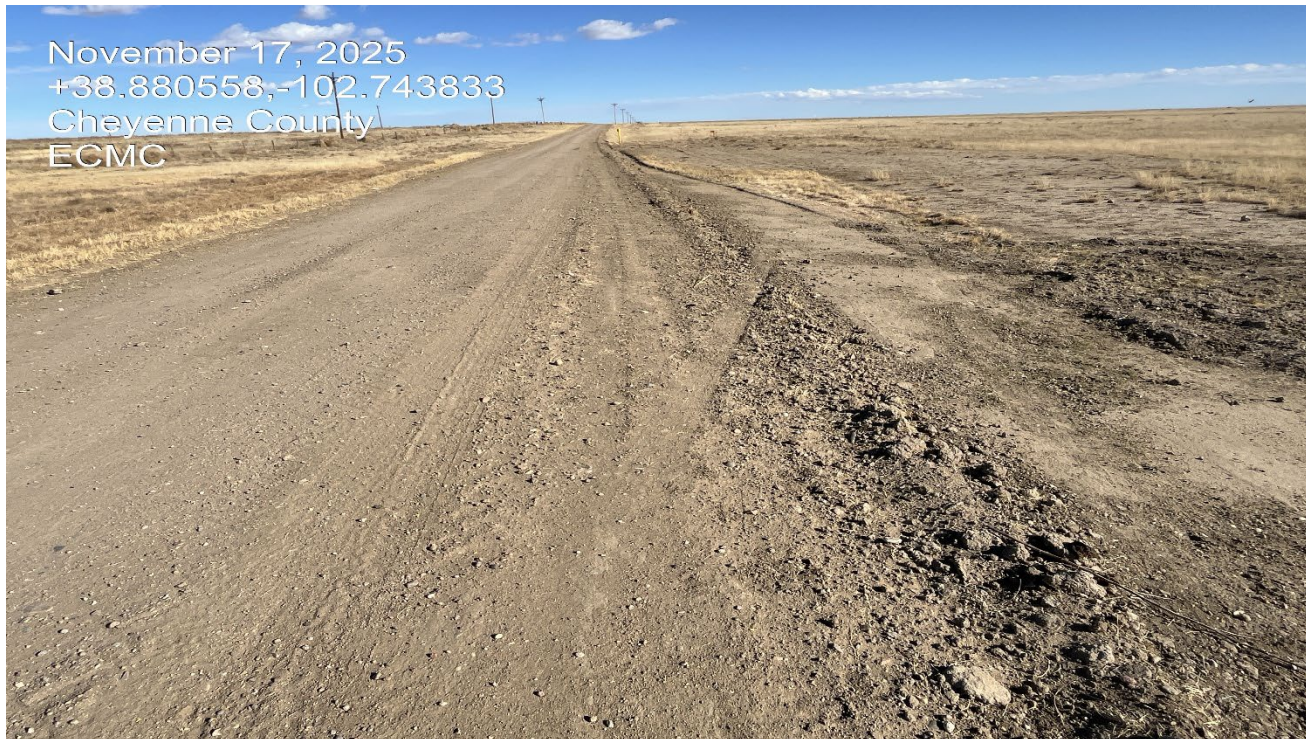
Photo 3. Facing east along the access road. The road has been regraded. The disturbed area where vehicles were driving will need to be decompacted and reclaimed.
