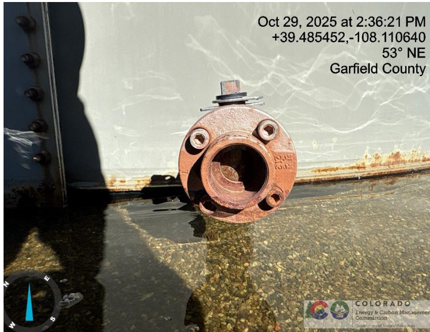
Photo # 3935 From inspection/audit 708907782 conducted on 10/29/2025 - Open ended load line
