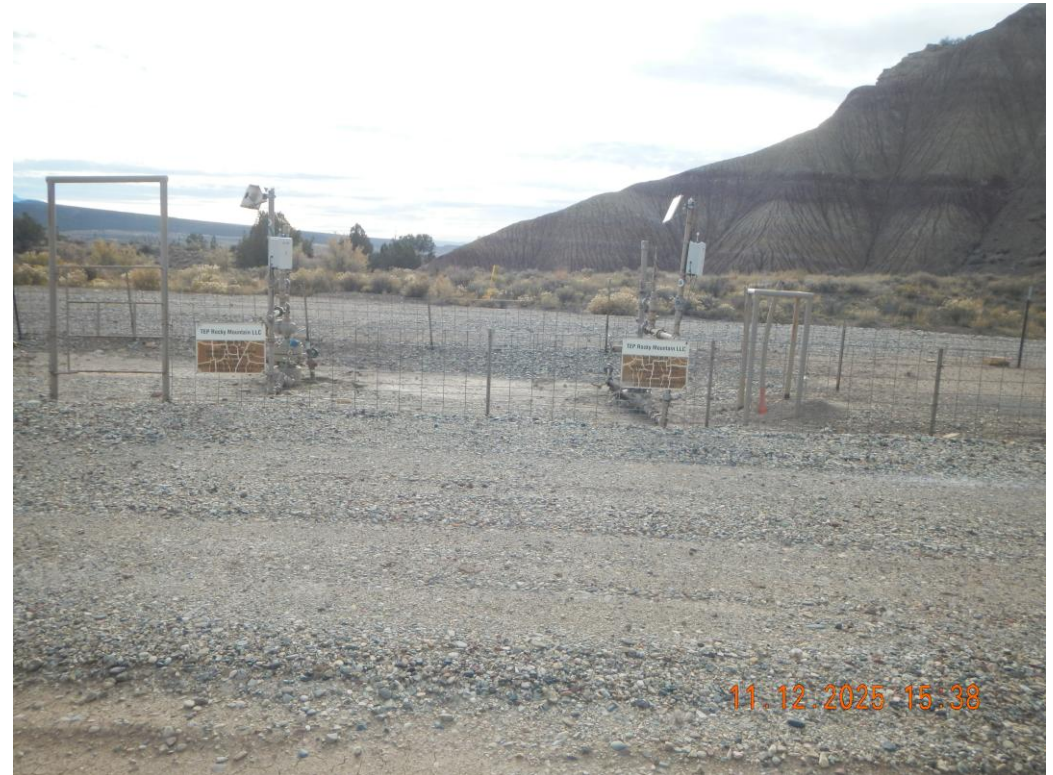
Signs are discolored and weathered.
