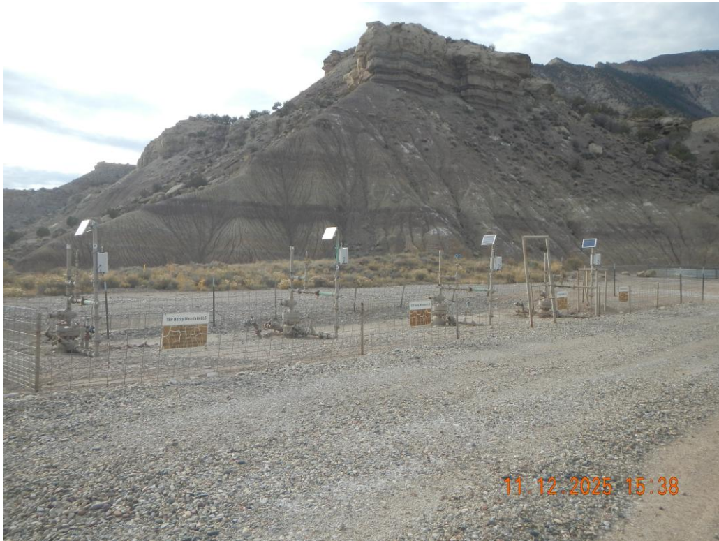
Signs are discolored and weathered.
