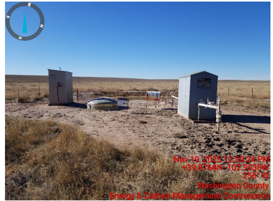
2. Meter shed, VGS shed and fiberglass tank
