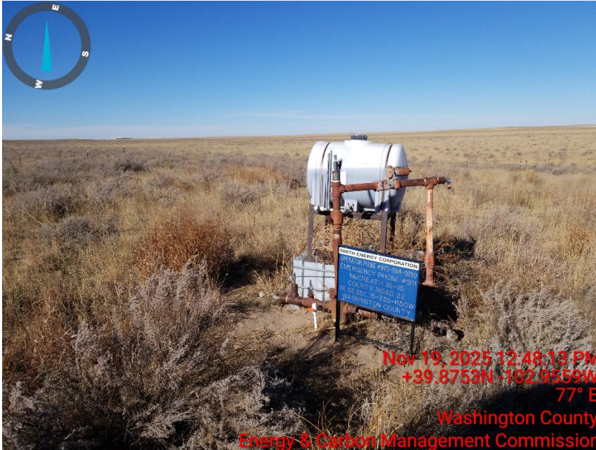
1. Wellhead and chemical tank
