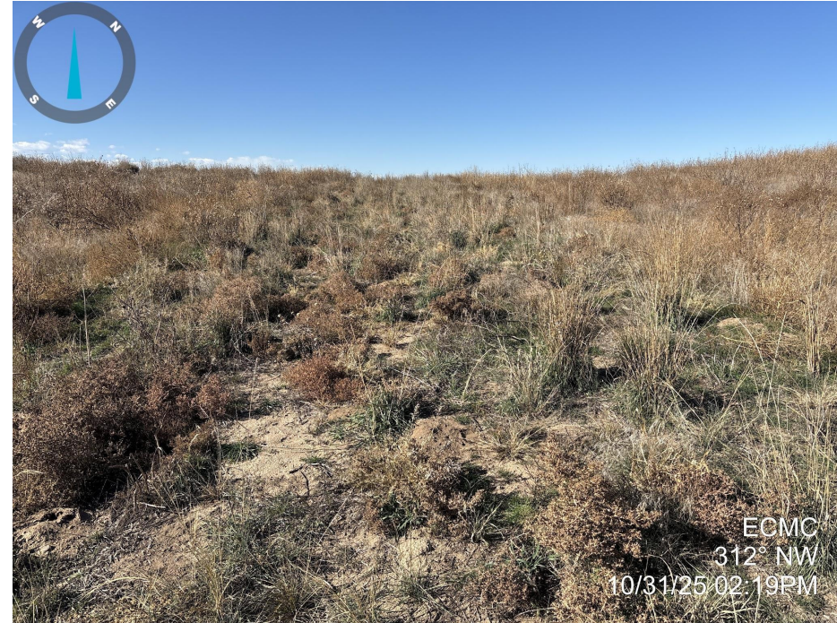
Photo 6. Photo taken of the access road to the multi-well location, facing northwest. Photo illustrates that the access road does not meet Rule 1004 standards.
