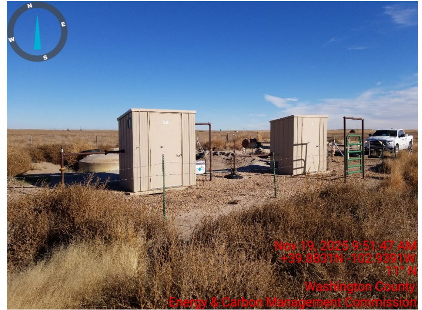
4. THIM 8-14 metal sheds
