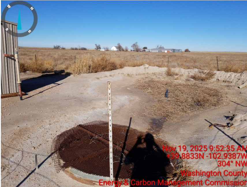
3. THIM 4-14 pit on east side of metal shed
