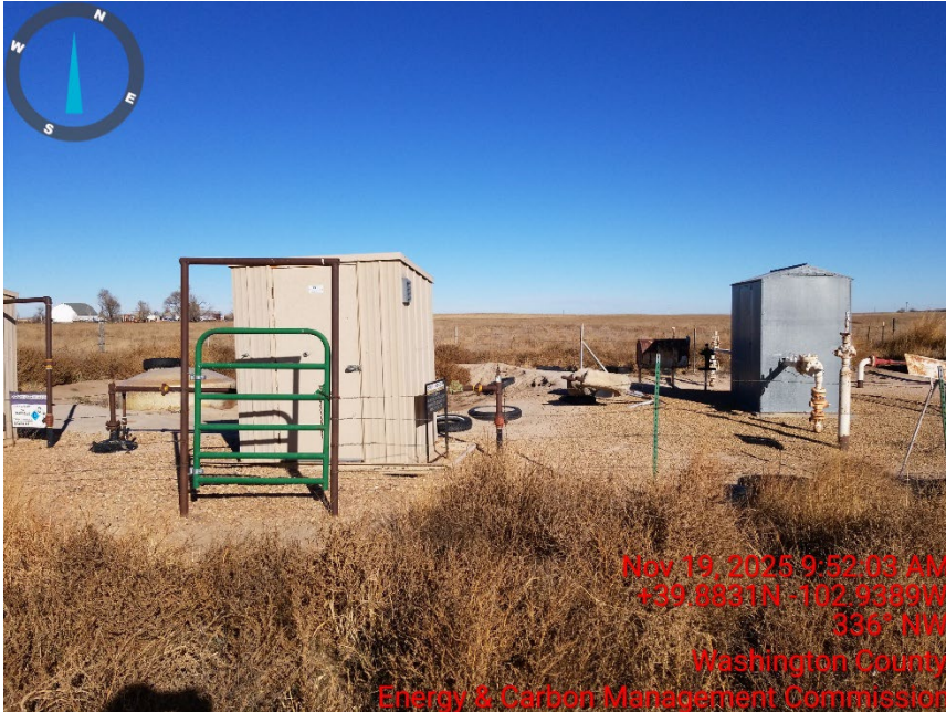
5. THIM 8-14 meter shed
