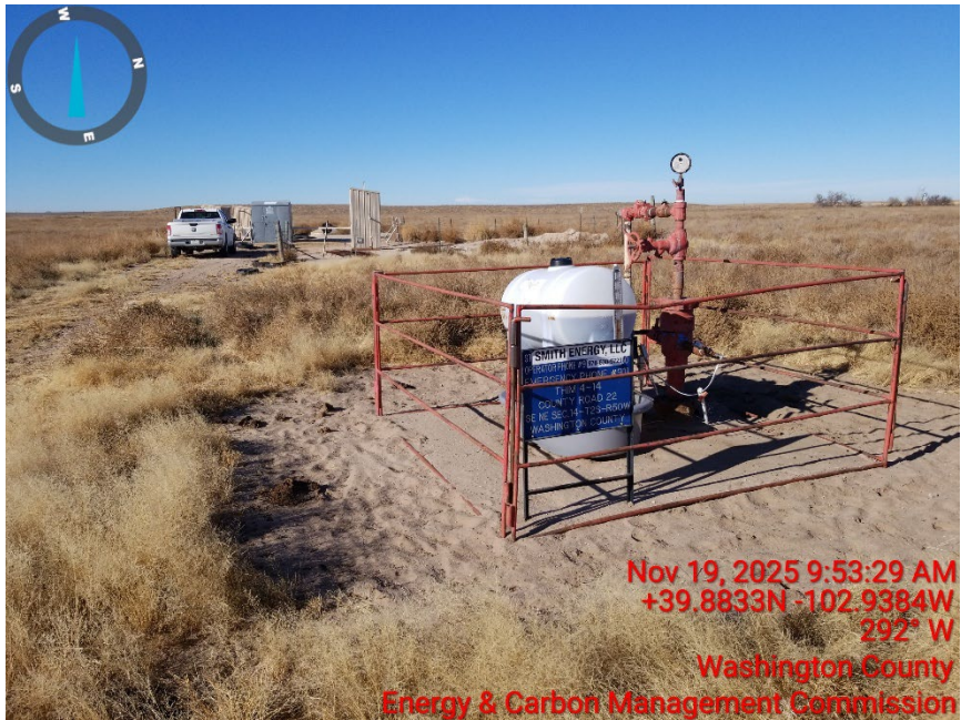
1. Wellhead and chemical tank
