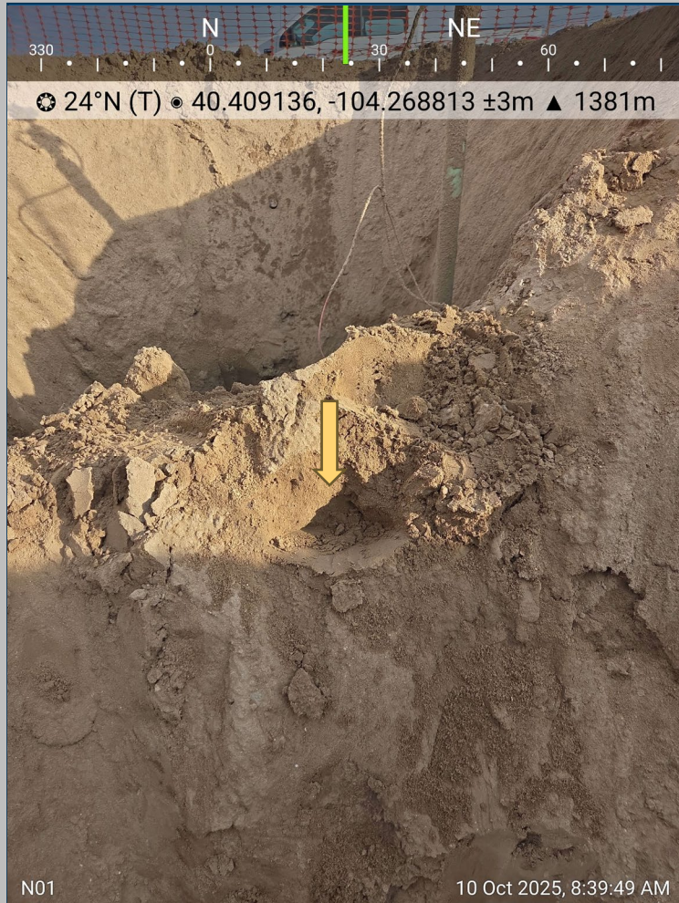
Wellhead North Sidewall Sample N01@3'
