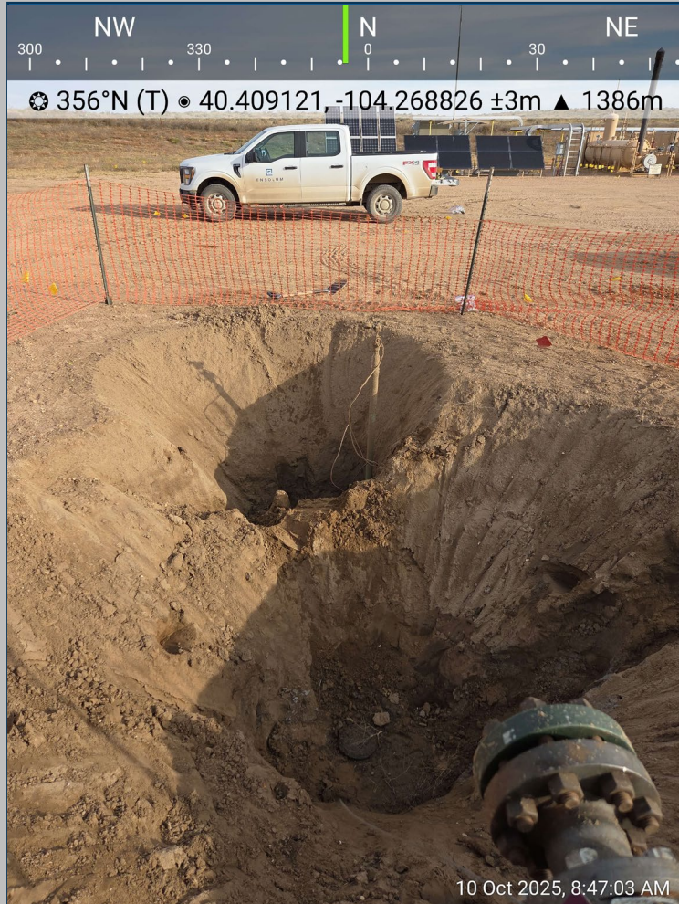
Wellhead Excavation Facing North
