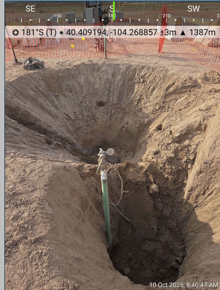
Wellhead Excavation Facing South
