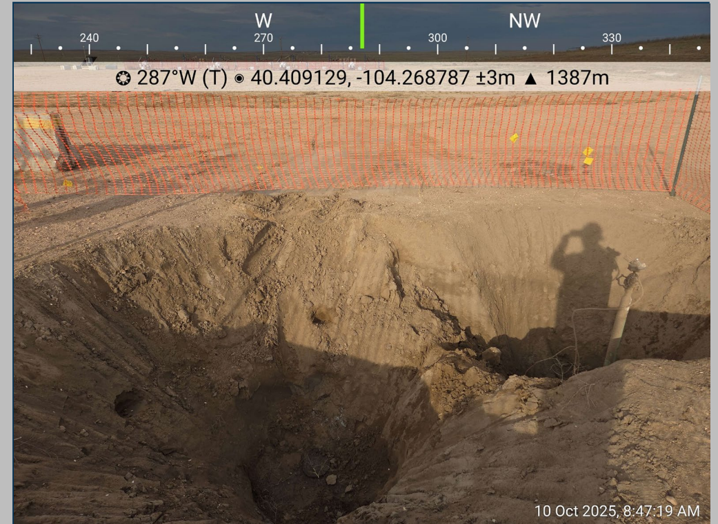
Wellhead Excavation Facing West
