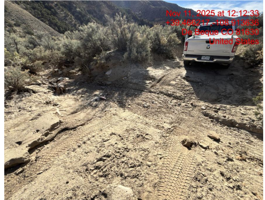
Lease Road Erosion – Photo #01535
